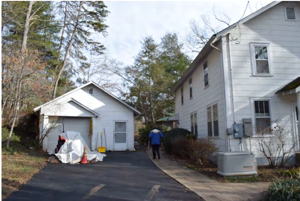
Alma and C. R. Thain garage, view to the east
