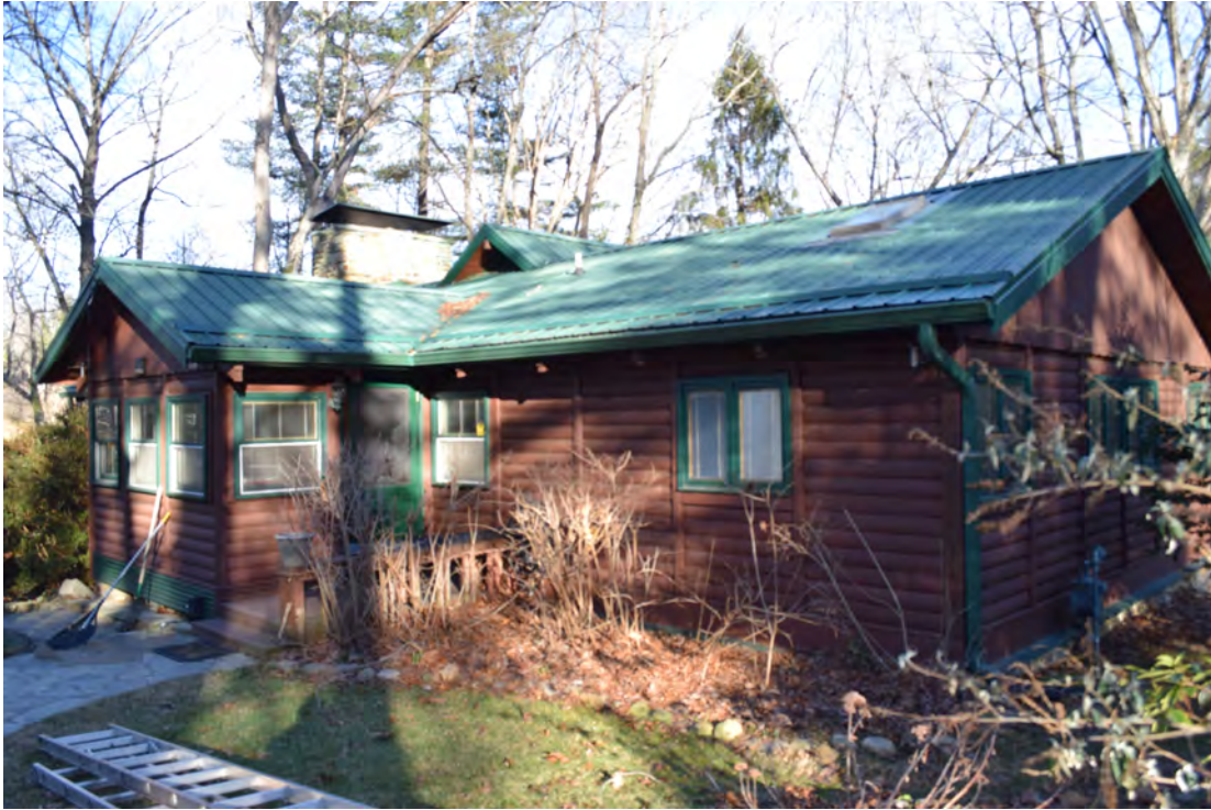
Doris and Edwin Brown House, view to the northeast
