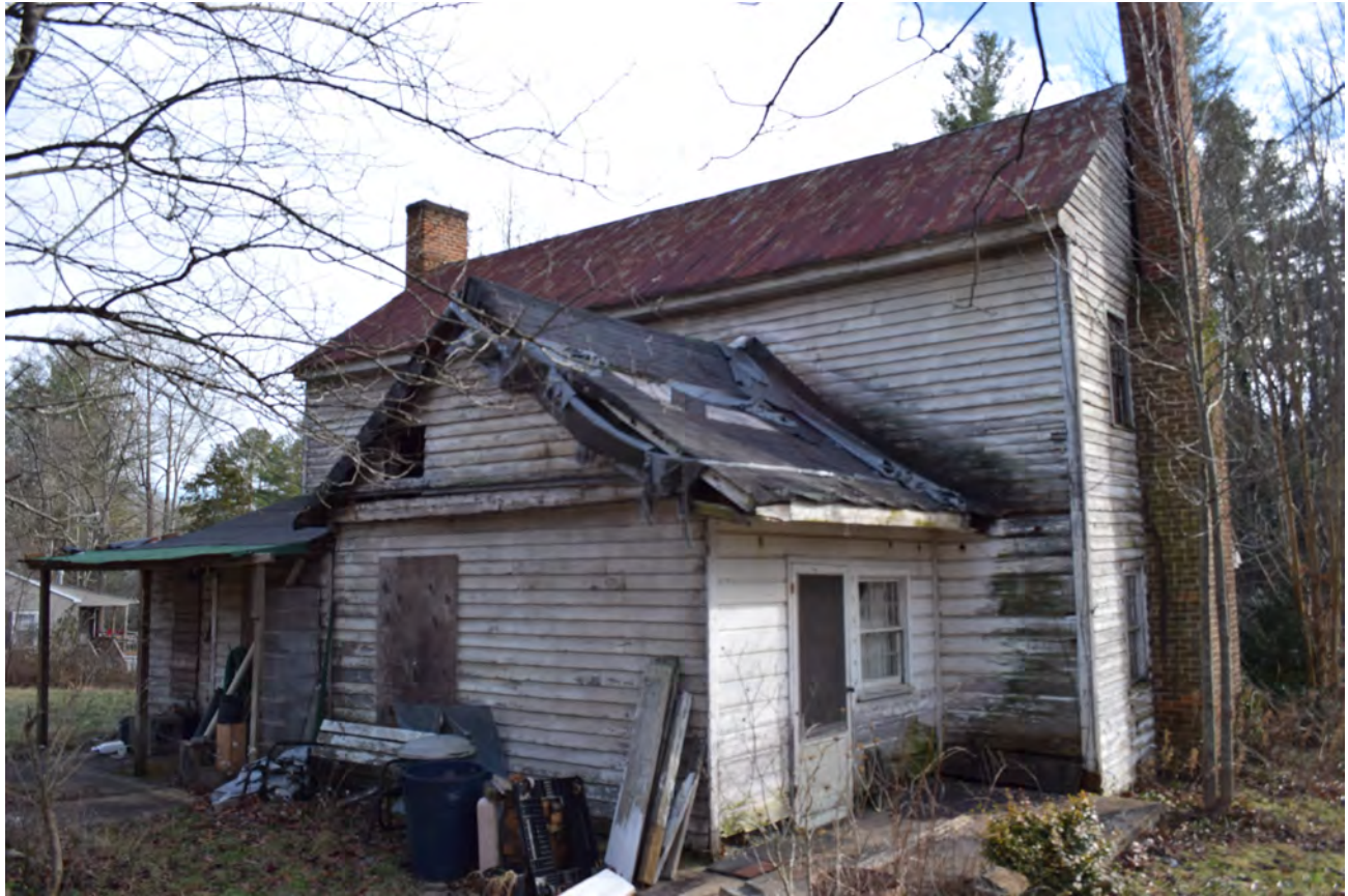
View of the rear elevation toward the southeast
