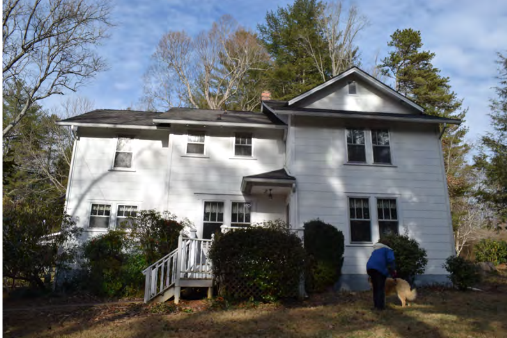
Alma and C. R. Thain House, view to the north
