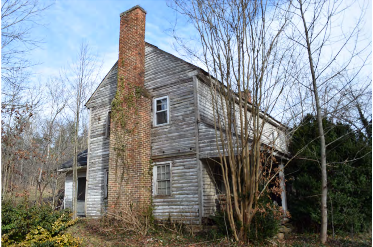
John Shroat House (BN0655), southwest corner, view to the northeast
