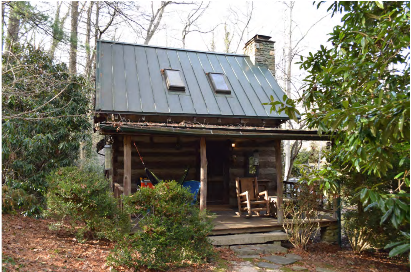
Facade of nineteenth century log house, view to the west
