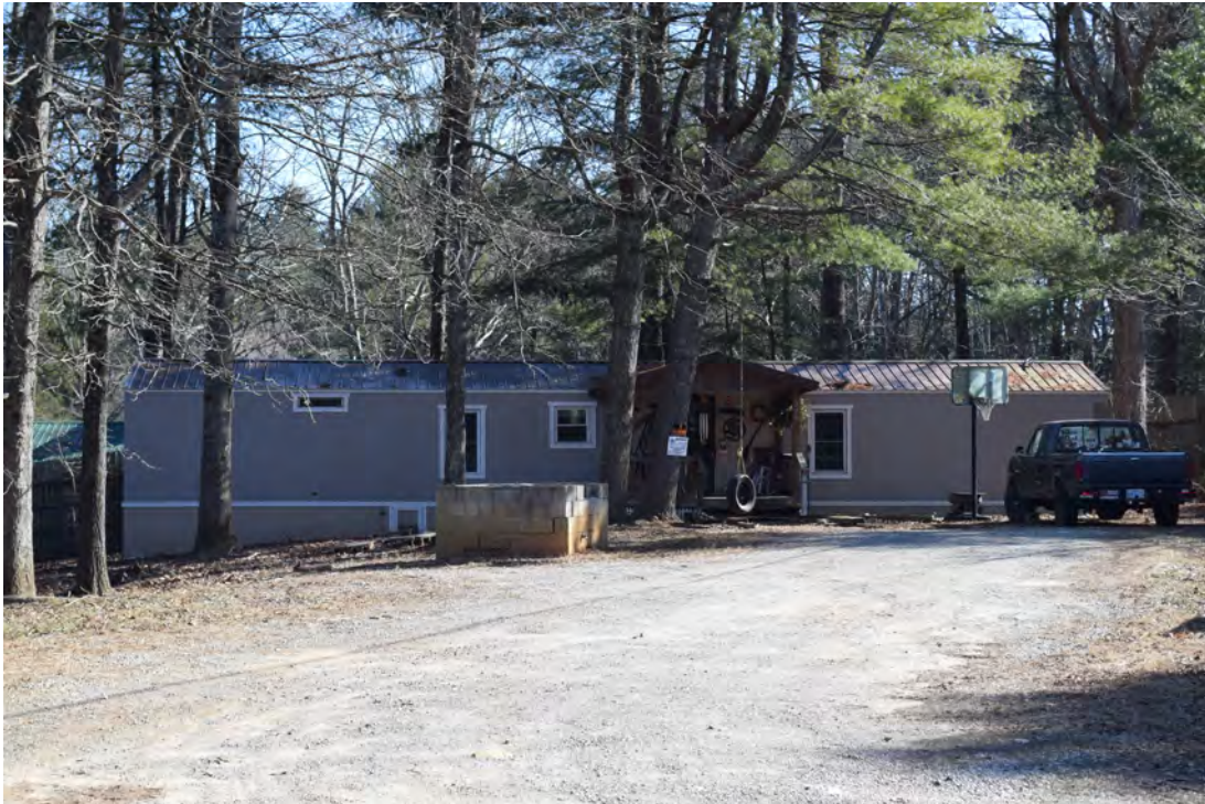
Single-wide mobile home on the Hare House parcel. view to the southeast
