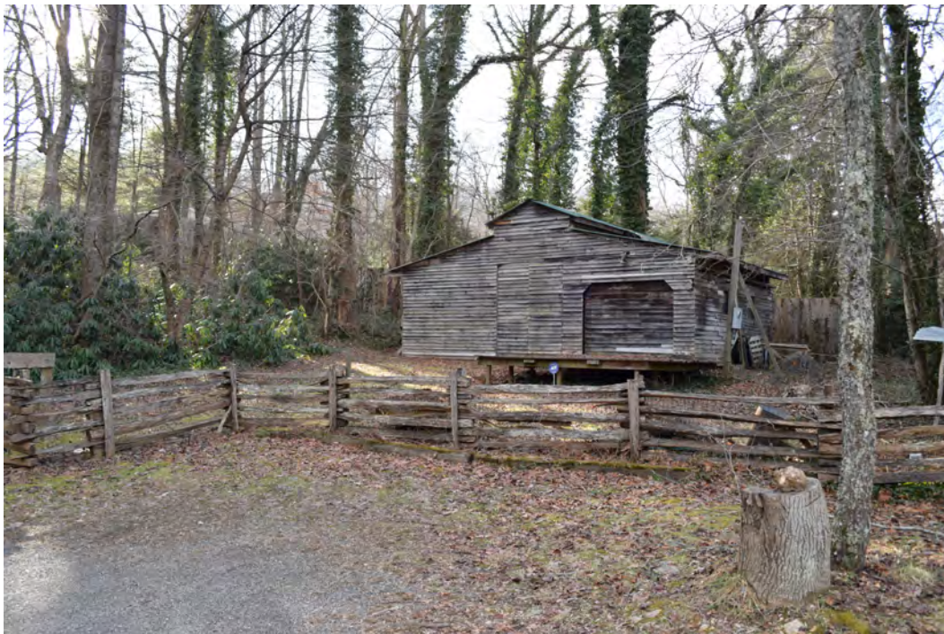
Barn behind house (BN6324), view to the west-southwest
